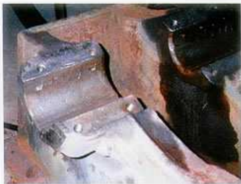
Left: A main bearing saddle prior to rebabbitting.
